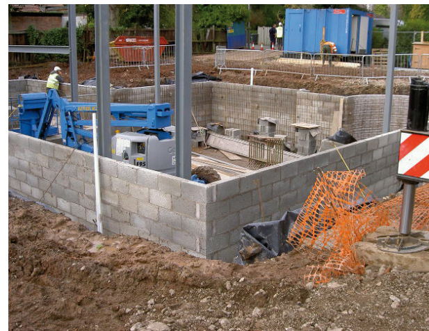
External block wall construction
