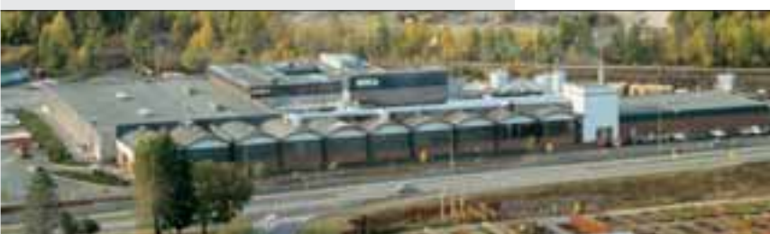
Isola Factory, Eidanger, Norway
