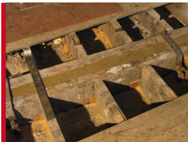
Beam strengthened with cured Trimol 36
