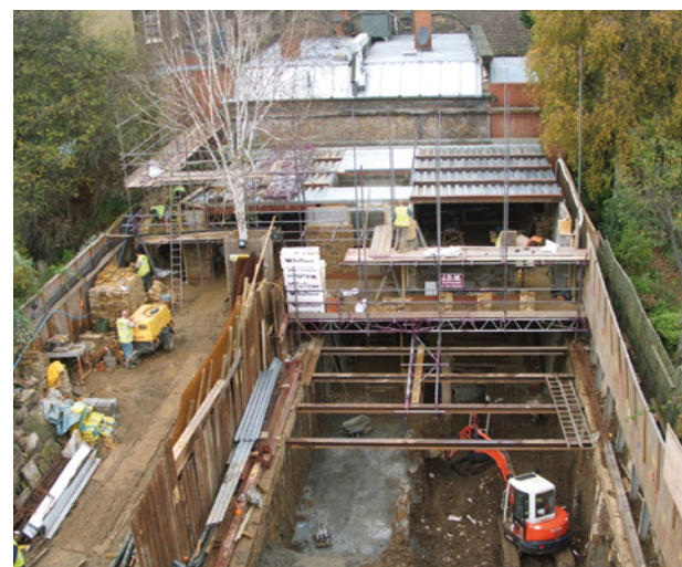
The new basement extends beneath the garden to the far end of the property
