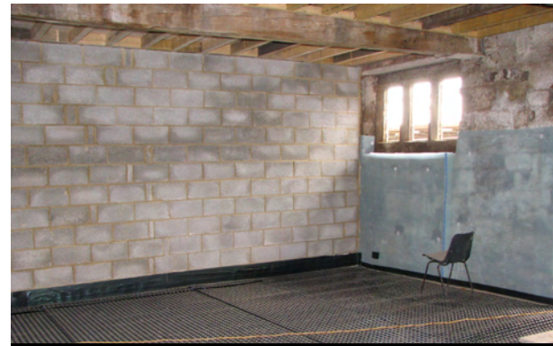
Platon membranes installed to internal walls and floors
