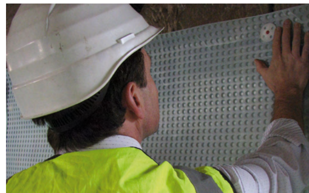
Cobb plugs were used to fasten the membrane in place of normal brick plugs
