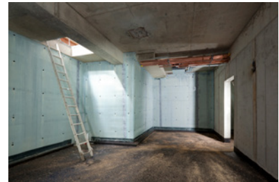
Existing Basement Waterproofing
