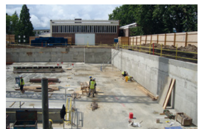
Type B Waterproofing
