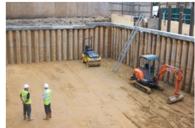
Watertight Concrete Basement in Construction
