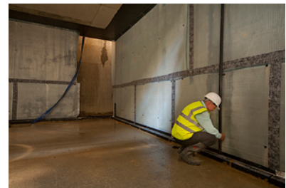
New Build Basement Waterproofing
