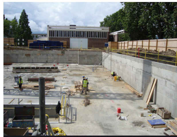
A completely watertight concrete system to floor and walls
