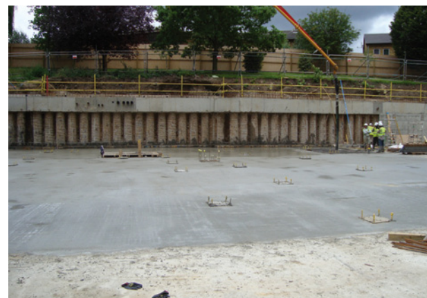
The 300ml floor slab was poured in three stages
