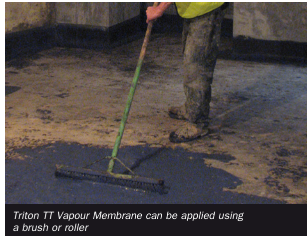
Triton Vapour Membrane is rapid drying, two coats can be applied in a day
