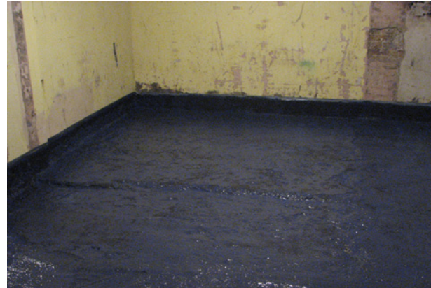
Triton Vapour Membrane is rapid drying, two coats can be applied in a day
